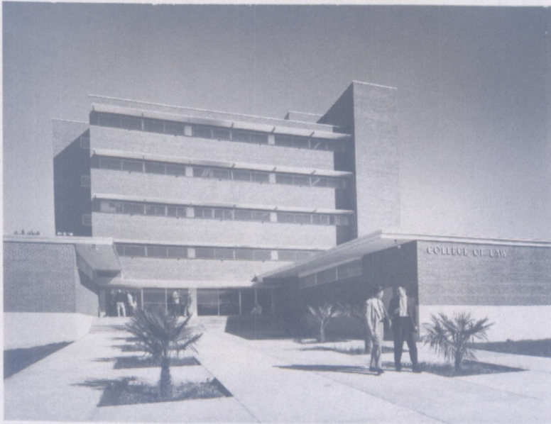
The Franklin Building was the College of Law's home from 1961–1979. (Manley Commercial Photography)
